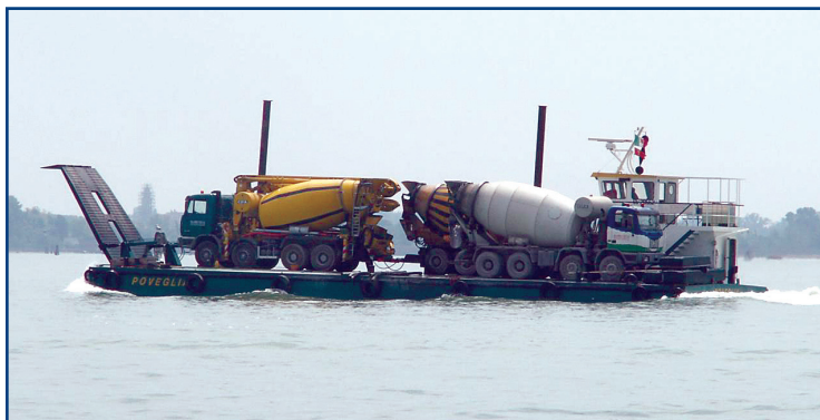
May be classified as "difficult construction access"? (From Venice.)
