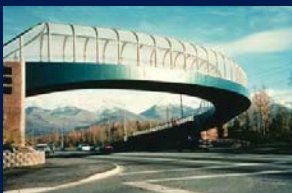
Tudor Road Bridge PND, Anchorage, AL
