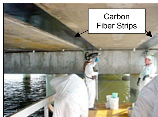
Figure 21: Bridge Strengthening [33]
