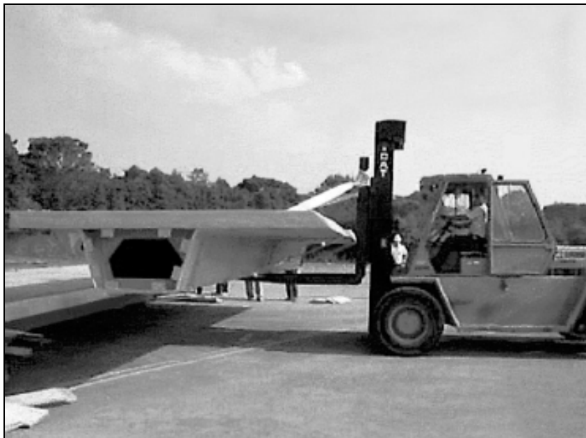
Figure 25: Element of composite bridge deck transported into position [38]
