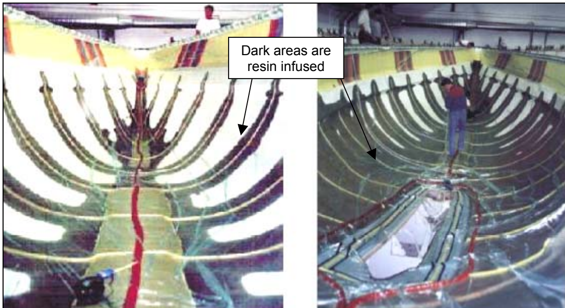
Figures 5a and 5b: 54 ft long fiberglass boat hull under vacuum resin injection [8]
