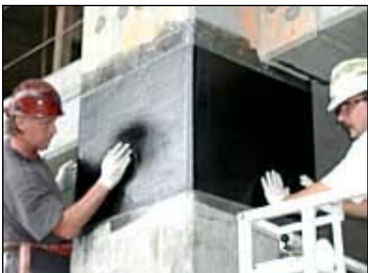
Figure 20: Column Strengthening [33]
