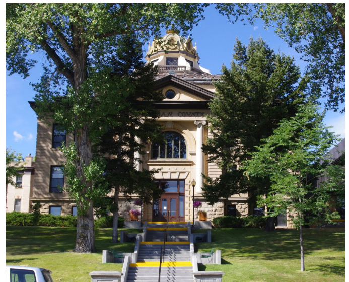
Figure 2. The historic Sheridan County Courthouse in Wyoming.
