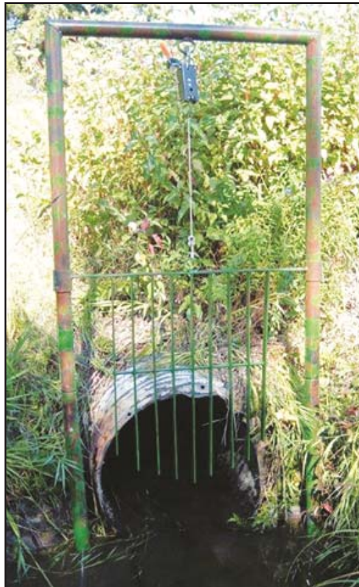
This photo shows the gate open with the use of the come-along in place, hoisting the gate.
