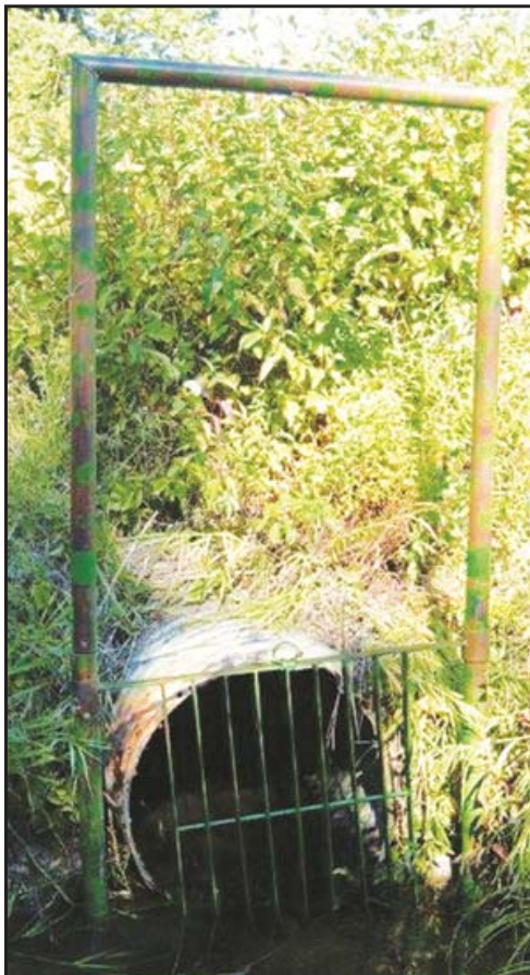
This photo shows the gate in a closed position over the culvert. (No come-along used when closed.)
