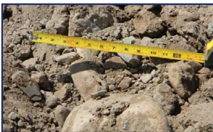
Above: Ripped Roadway Gravel
