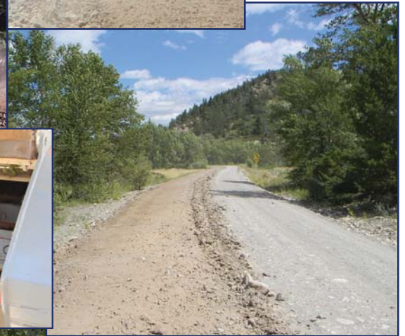
Above: Crushed roadway gravel on left-hand side after one pass with PTH Crusher 2500HD
