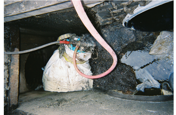
Polymer Culvert Lining During Curing
