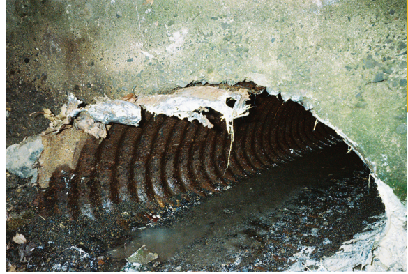
Deteriorated Culvert
