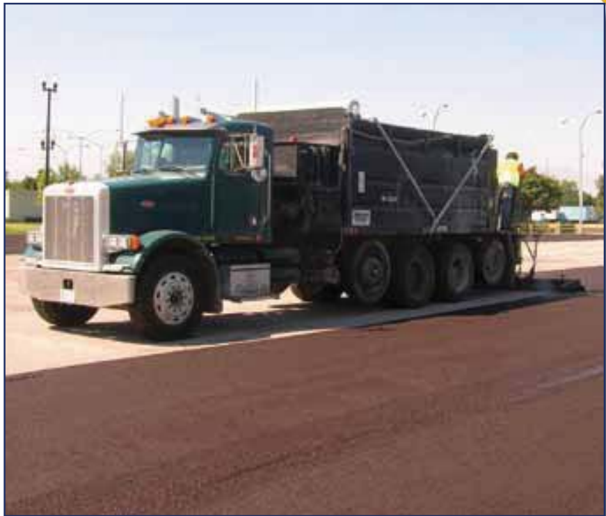
Used here in a parking lot, slurry sealing is an effective treatment to increase pavement life by up to seven or more years
