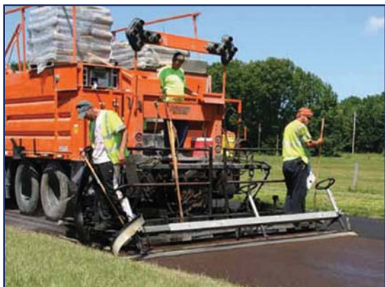
Just outside of Rockport, Indiana, micro surfacing treated an 8.5 mile stretch of S.R. 70 to improve skid resistance, increase wear life and correct minor rutting and surface deterioration
