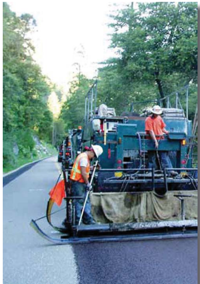
More than 2,287,000 square feet of Type III microsurfacing preserved 15 miles of U.S. Route 76 just north of San Diego, Calif. Photo courtesy of Bergkamp
