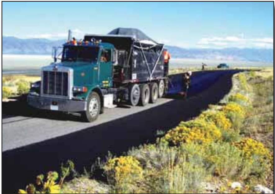
Micro surfacing is an environmentally safe application that leaves an aesthetically pleasing black surface and minimizes life-cycle costs Photo Courtesy of Bergkamp
