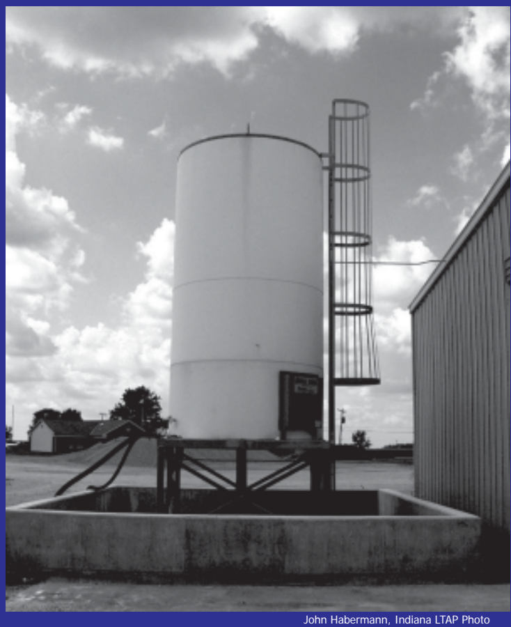
6,000 gallon tank with poured concrete retaining system
