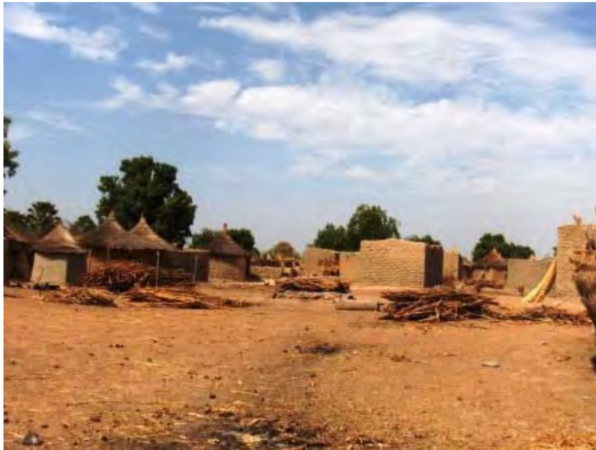
Figure 5. Sanambele village buildings. Note that they are made of clay bricks with thatched roofs. (Dunkel, 2009).
