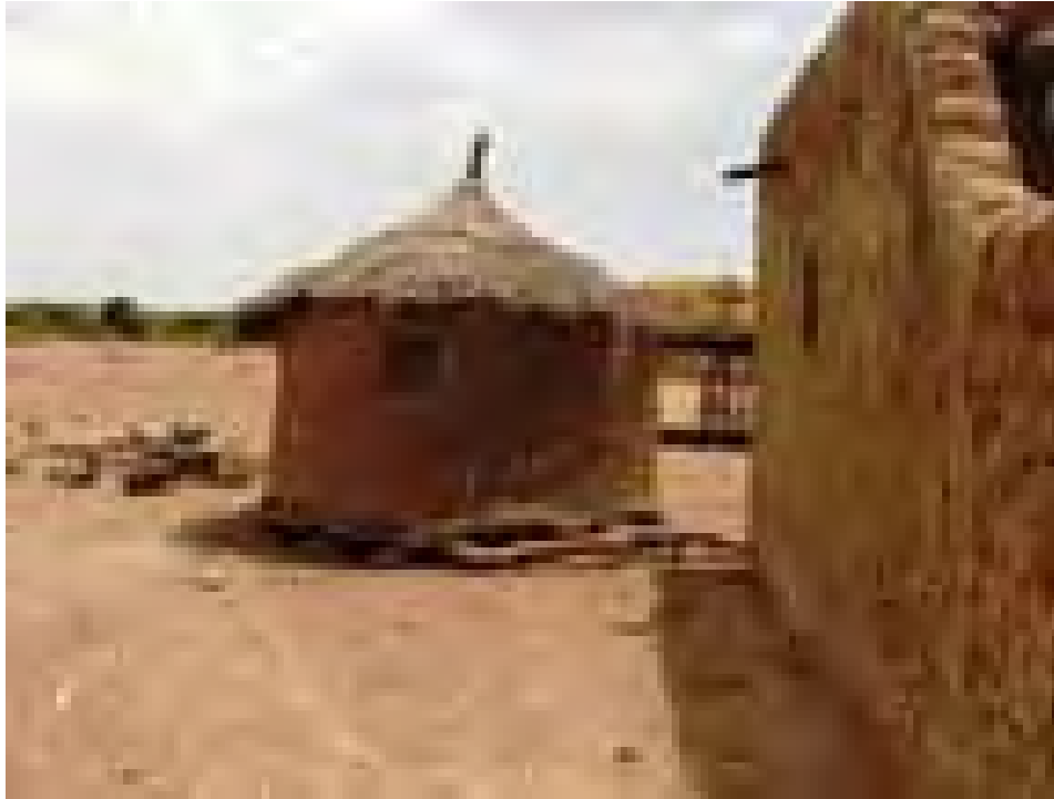
Figure 6. Gigne, a Sanambelean grain storage facility. (Dunkel, 2009).
