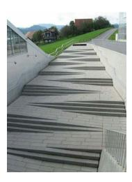
Inclusive Design can produce a single solution by integrating features to address the needs of diverse user communities. For example, this staircase integrates steps with ramps for access by
