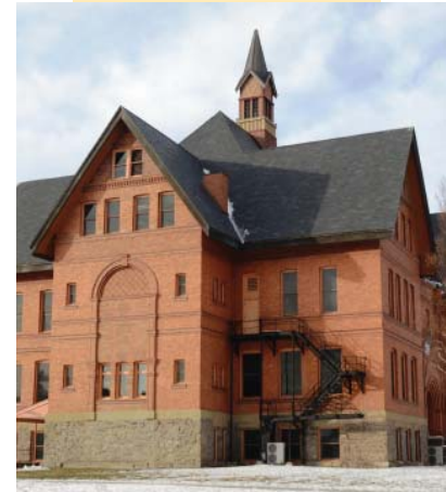
New cupola on Montana Hall
