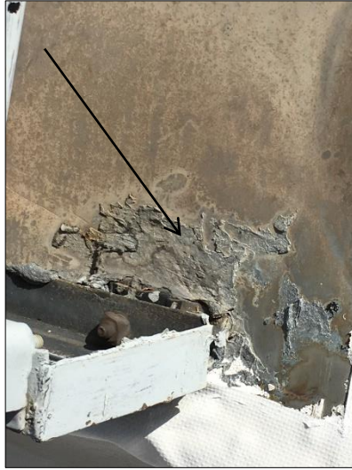
Silver Tar Coating on Mechanical Unit
