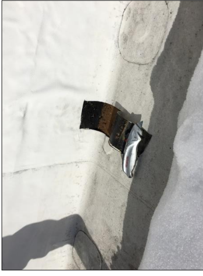
Stairwell Roof Parapet Wall Sample
