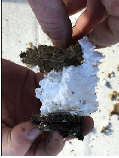
Upper Main Roof Core Sample
