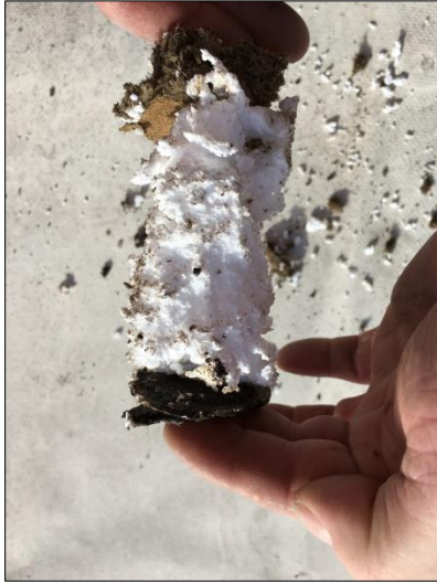
Lower Roof Core Sample
