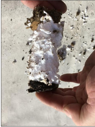
Lower Roof Core Sample
