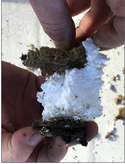
Upper Main Roof Core Sample
