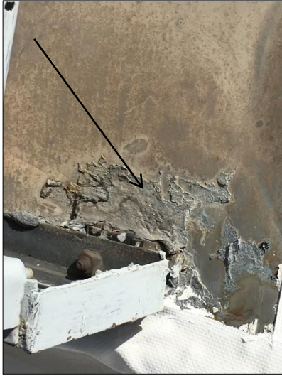
Silver Tar Coating on Mechanical Unit
