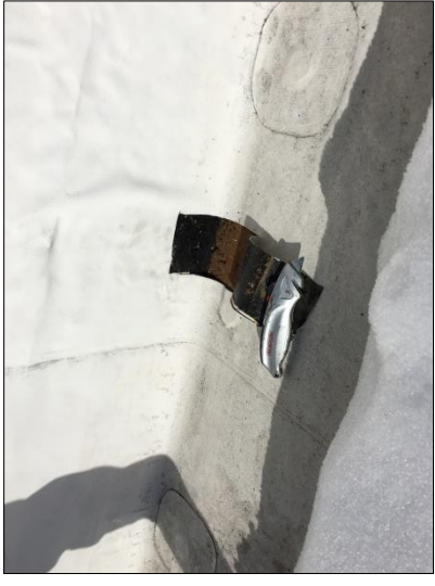
Stairwell Roof Parapet Wall Sample
