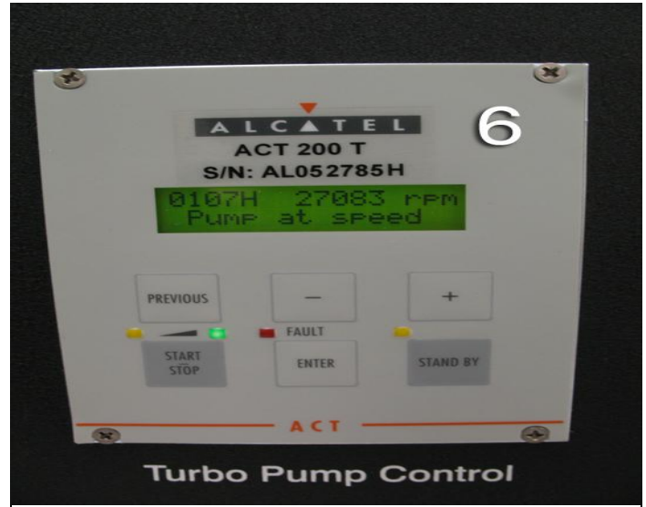
Above: Turbo Pump Control fully ramped
