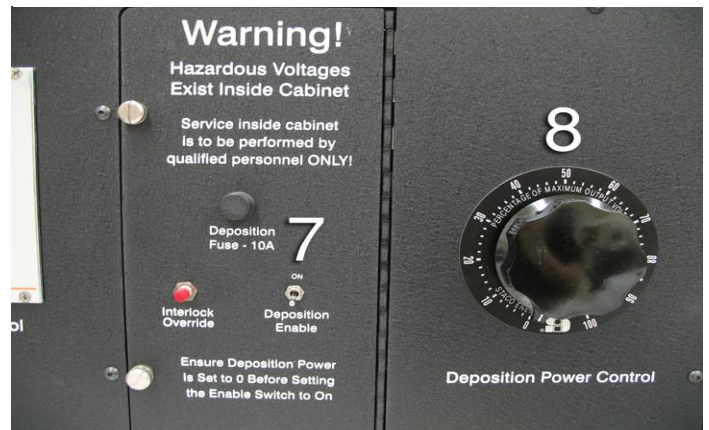
Above: Deposition Controls
