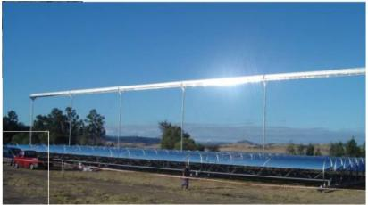
Figure 50: Fresnel Lenses at Liddell power station used for hot water heating Image Source: Morrison G.L. (2003), *Solar Thermal Electricity* [online], Available: <u>http://solar1.mech.unsw.edu.au/glm/clfr/solar%20thermal%20electricity.htm</u> (Accessed 21st June, 2007)
