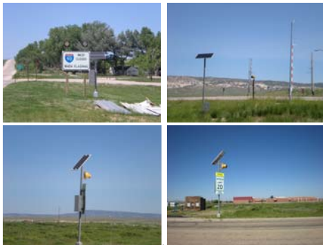
Montana State University: Solar Cells Lecture 9: PV Systems 9
