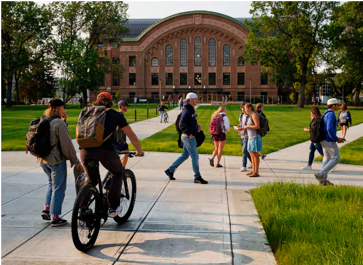
Romney Hall has been undergoing extensive renovations and will reopen in November 2021
