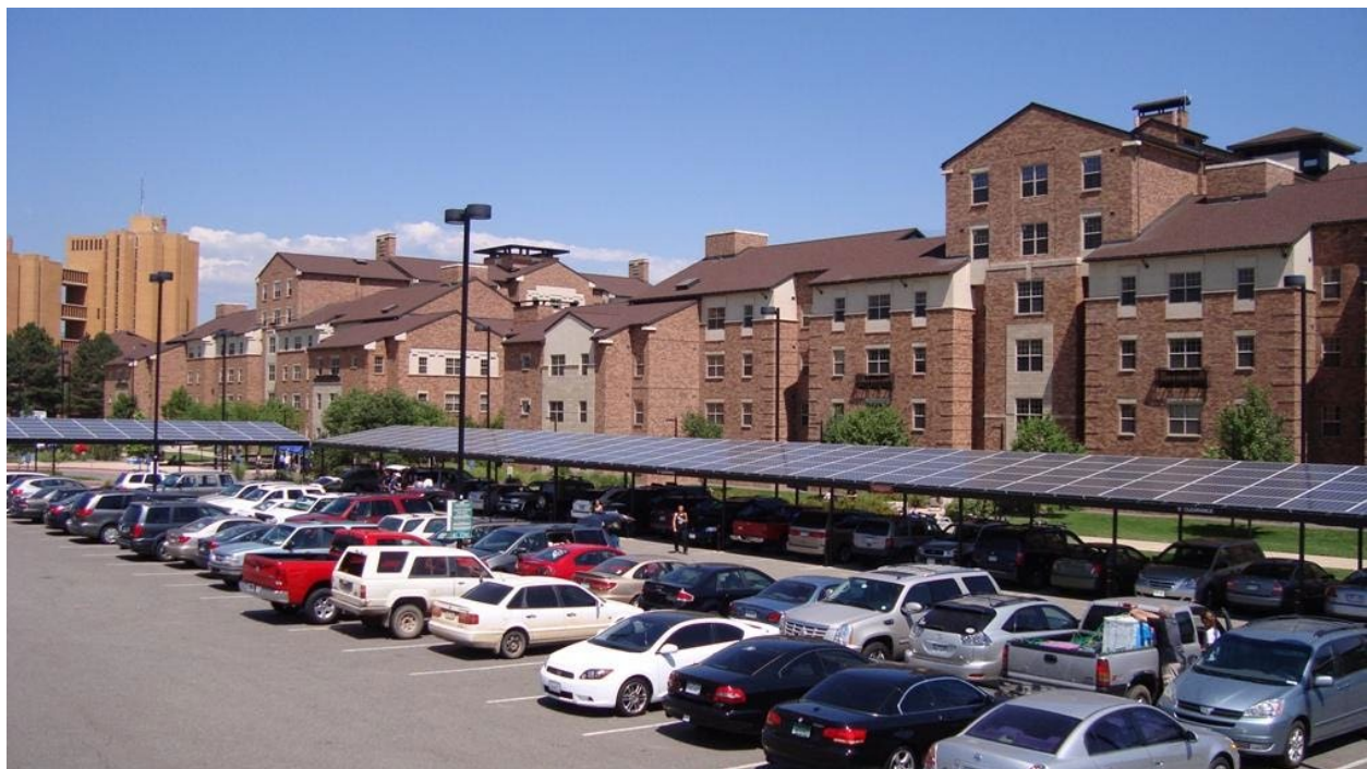
Figure 2: CU Boulder Solar Carport
