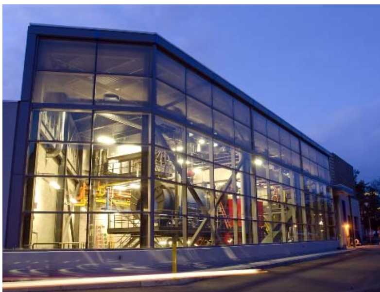
The new biomass-fired power plant at Middlebury College in Vermont (Photo credit: Brett Simison)
