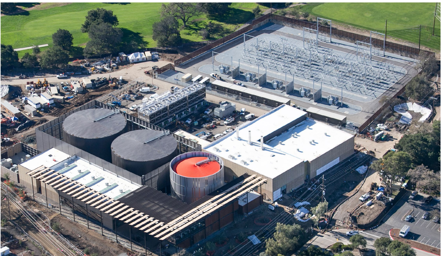
Photo: SESI represents a transformation of university energy supply from 100 percent fossil-fuel-based combined heat and power plant to grid-sourced electricity and a more efficient electric heat recovery system
