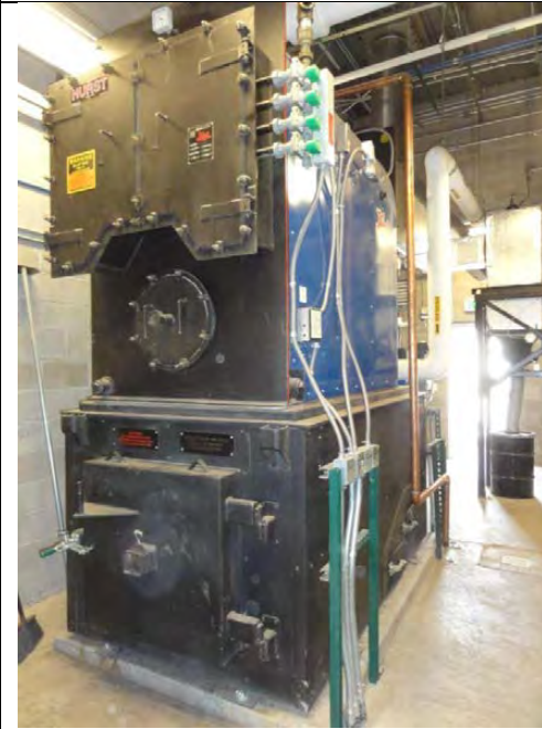
A. Small Institutional Boiler with typical efficiency of 70%. (Messersmith Mfg.)
