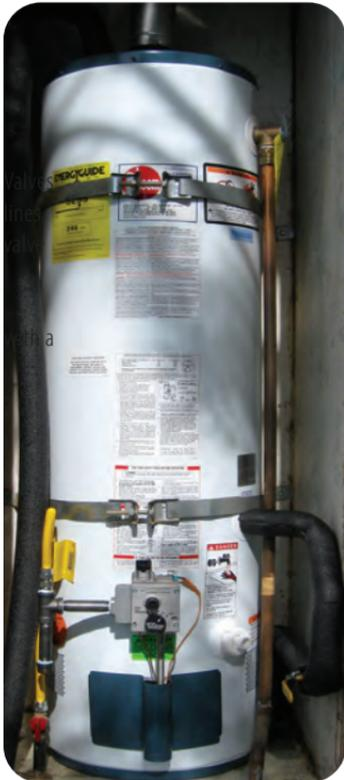
**Typical Water Heater.** This is nice clean installation. There is no evidence of rollout or scorching. Earthquake straps have been installed. Valves are installed on both hot and cold water and all the lines are insulated. The pressure relief (PRV or TP valve) has an extension to send any discharge to outdoors. The gas supply line is composed of black pipe and approved flex lines, drip leg to catch any condensation or debris.
