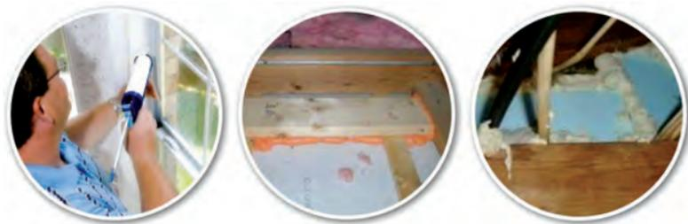
**What to Use for Air-Sealing.** Caulking, liquid foam, and sheet goods that include foamboard, drywall, and plywood. These are the most common materials for air-sealing, and you'll be most productive if you have plenty of them on the truck at all times.
