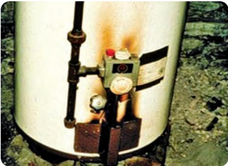
**Evidence of Rollout.** This water heater has plenty of evidence of poor draft: scorching from rollout, and corrosion caused by the condensation of escaping flue gases. This is surely a fire hazard, and could be a health hazard if the appliance is spilling combustion gasses. Do not take these signs lightly—people die every year because of poorly maintained combustion appliances just like this.
