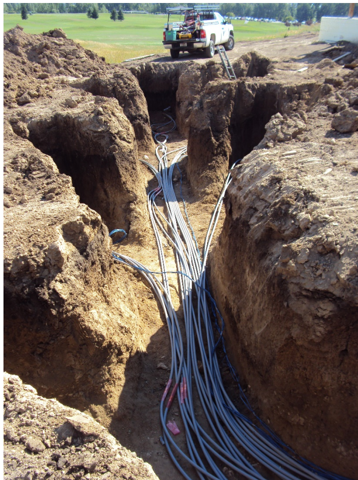
Figure 11. Trenching works towards the house
