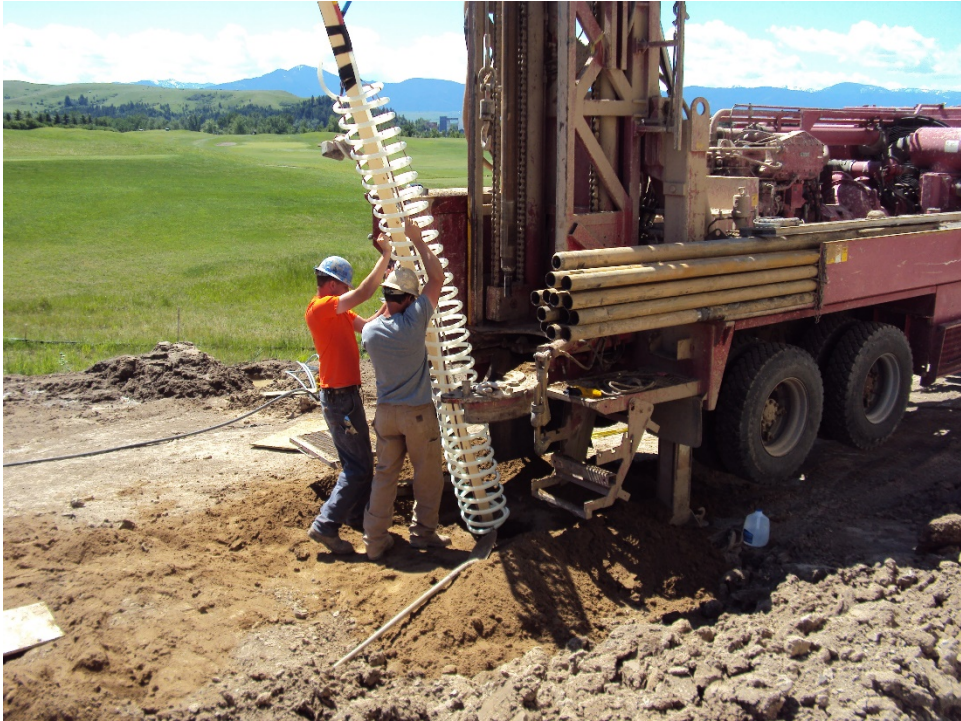
Figure 9. Installation of a helix probe
