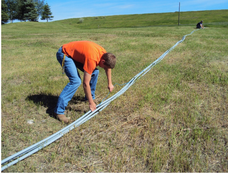
Figure 10. Sensor installation on a vertical 2-U bend probe with spacers.
