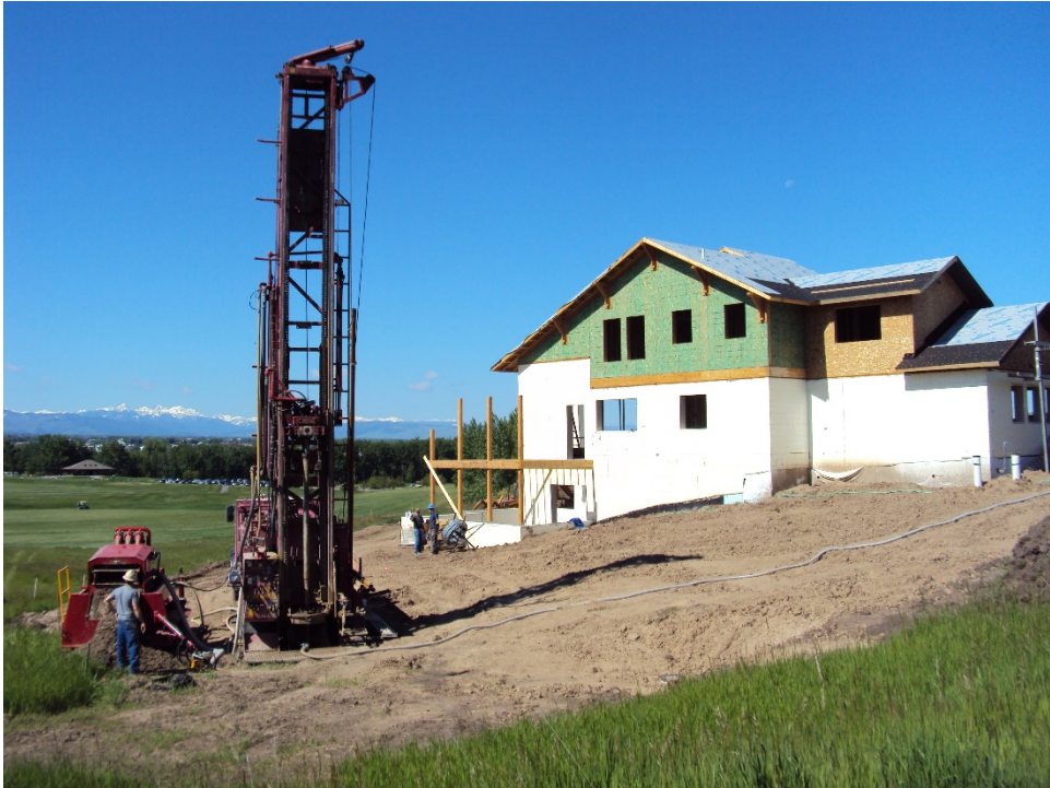
Figure 8. Drilling operations during construction
