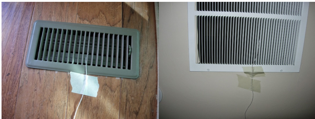
Figure 6. Floor Register and Return Grille
