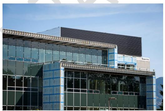
Figure C-12: View of the Transpired Solar Collector at Jabs Hall, Bozeman Montana Central Equipment:
