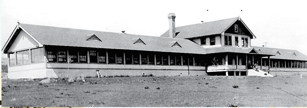
Sleeping pavilion at the Montana Tuberculosis Sanitarium. Photo courtesy of the Powell County Museum, Deer Lodge
