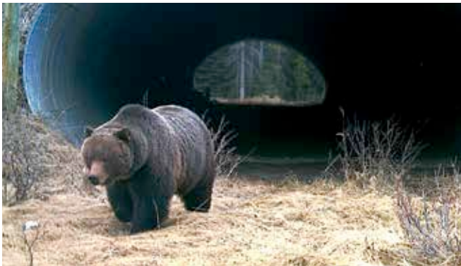
A radio collared grizzly passes through an underpass at Castle Junction below the Trans-Canada Highway in Banff National Park. Photo courtesy of HighwayWilding.org.
