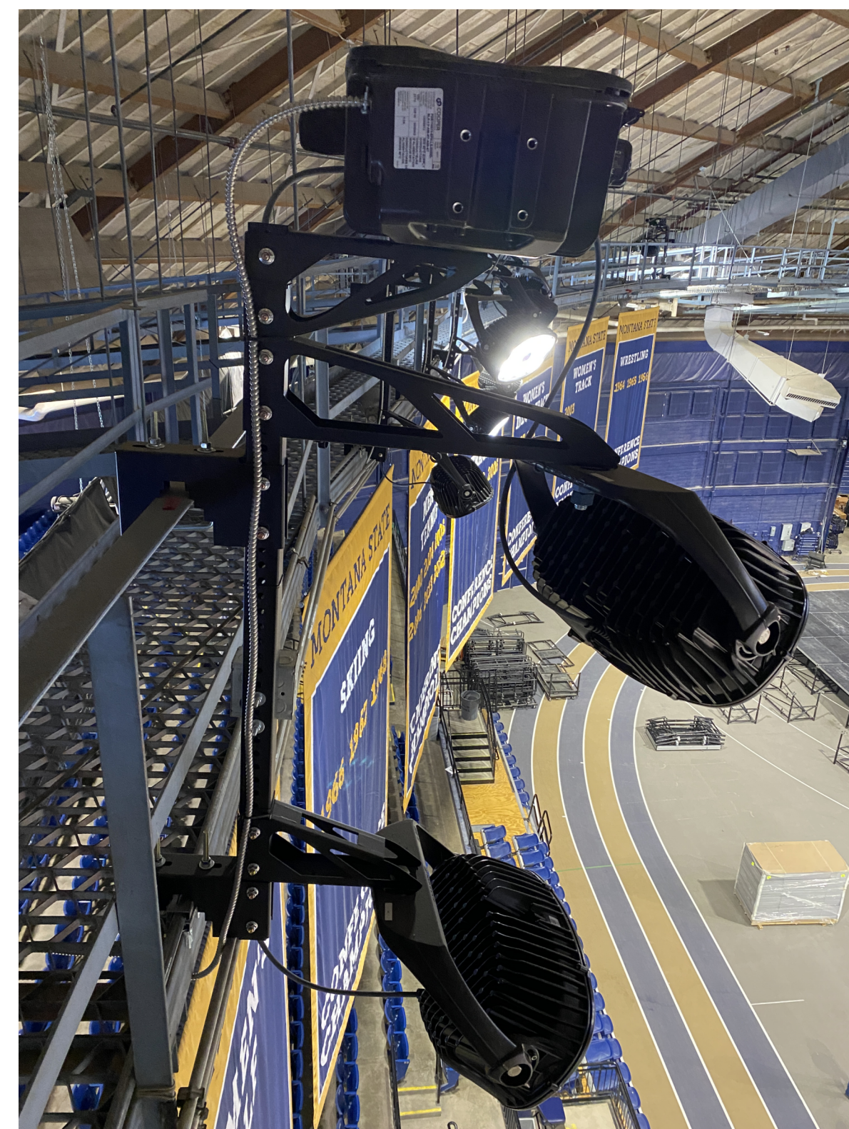
2 LUMINAIRE TYPE B01 EXISTING MOUNTING CONDITION PHOTO ELO.01 1/4" = 1'-0"
