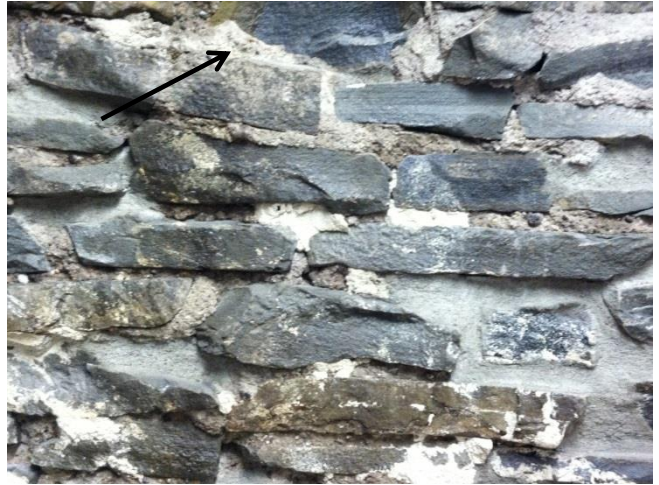
Foundation Rock Pointing (Mortar)
