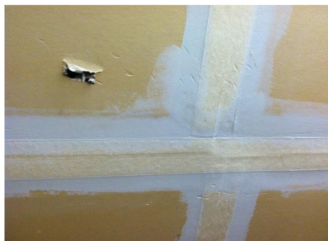
Drywall / Mud / Texture
