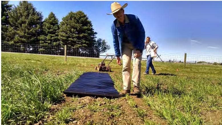
Picture 4. Level and compact the soil under the pipe track. Roll out landscape fabric and place the pipe track on top of the fabric. The fabric will keep the weeds down and help keep the casters out of the mud.
