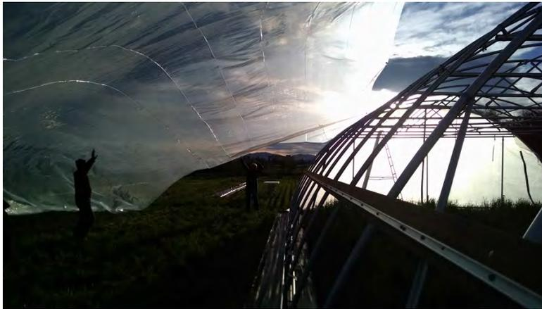
Picture 10. The remaining crew members lift the film so that it doesn't snag on the frame as it is being pulled.
