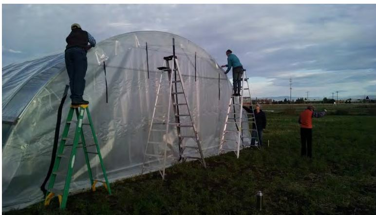
Picture 11. Plastic film is attached to one end wall then pulled just enough to get the wrinkles out of the film. Poly lock holds the film to the greenhouse without penetrating the film. The film is attached to the hip boards with poly lock and the bottom edge of the film is attached to the roll up side wall system.
