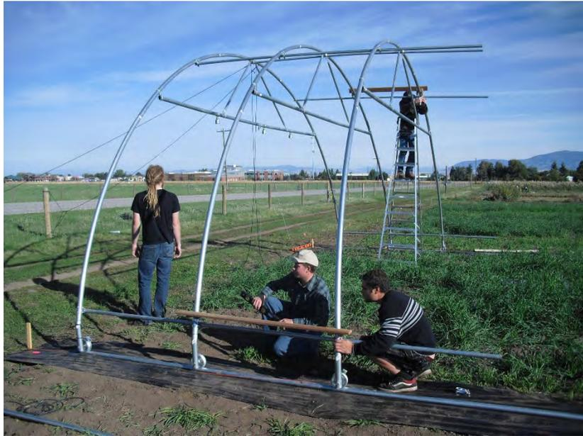
Picture 6. Note the two wooden jigs that were constructed to aid in spacing the arches on four foot centers. We built three spacing jigs and they were very helpful in the construction process.
