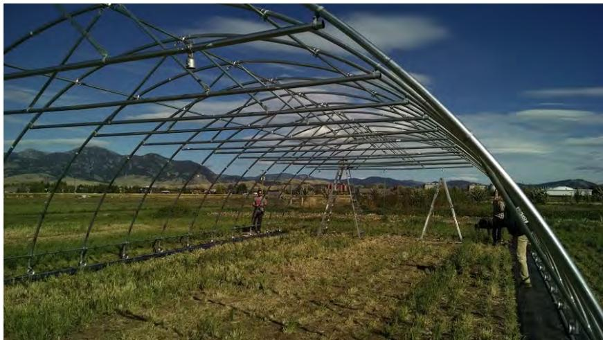
Picture 8. The arches are complete and the end wall framing is next.
