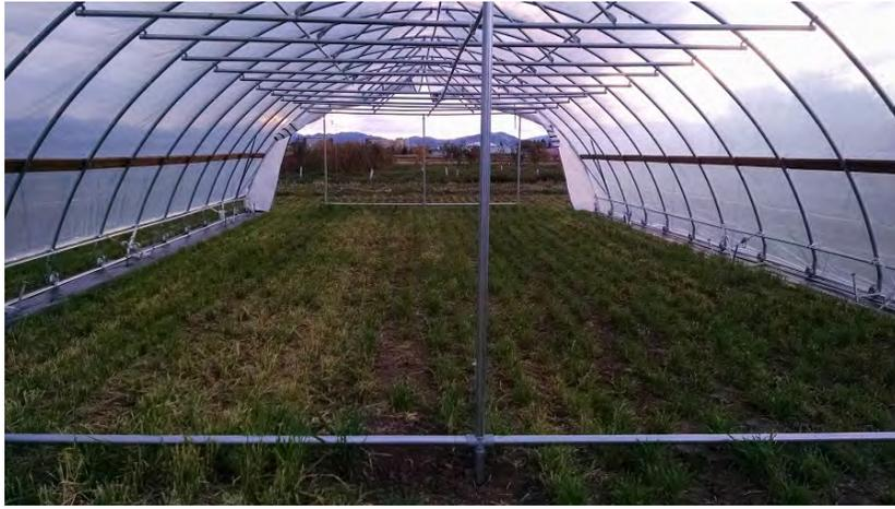
Picture 12. The completed moveable high tunnel. Casters at the base of the hoops are visible as are the stakes and straps that attempt to hold the tunnel in place. End walls are fully open and secured with straps.
