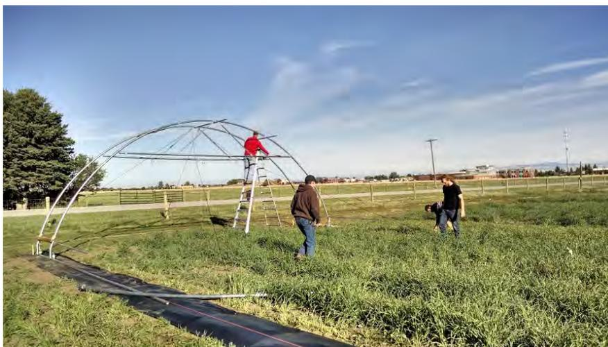
Picture 5. Setting the first two arches requires temporary bracing to hold the arches in place while fastening the purlins. Unlike a traditional tunnel that utilizes ground posts, moveable tunnels are not attached to the ground. With the first tunnel we used rope and ratchet straps to hold the arches in place, but it proved difficult to use. Subsequent tunnels used fixed bracing to hold the arches.
