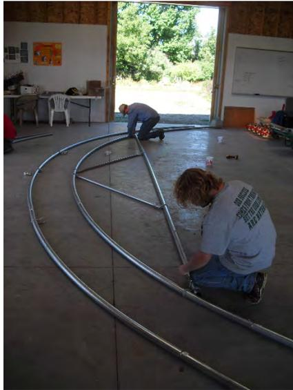
Picture 3. Assemble hoops on a flat surface which will aid in having the hoop and truss assemblies square.
