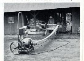
THE ELECTRIC PUMP.—It fetches water without grumbling, can serve all needs of the farm and home for about 25 kilowatt-hours per month.
